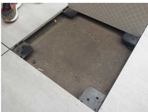
5: dakbedekking is droog tpv 'probleemgebied'
